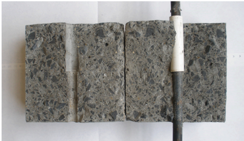
Fig. 5. Specimen after splitting cut along reinforcement bar.
