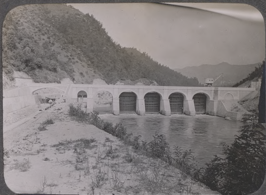
38. Robiate, Wehr m. Wehrkanal.
