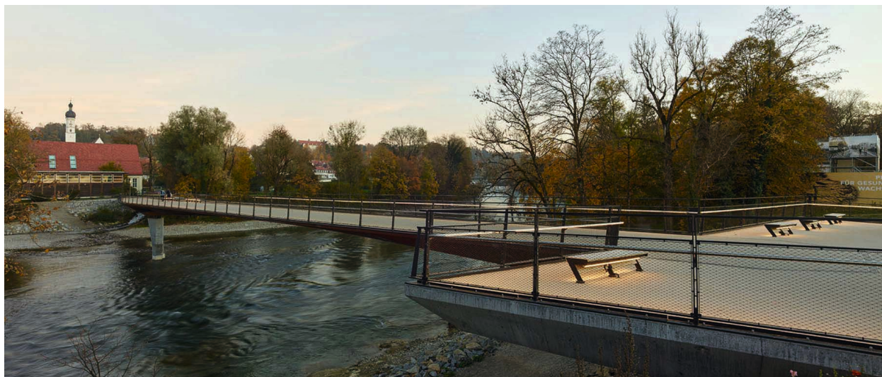
III. 7. 'Lady Herkomer Steg' in Landsberg on the Lech River, Germany, arch. Mayr-Ludescher. DKFS photo, source: https://dkfs.io/portfolio/lady-herkomer-2/ , (access: 02.02.2024)
