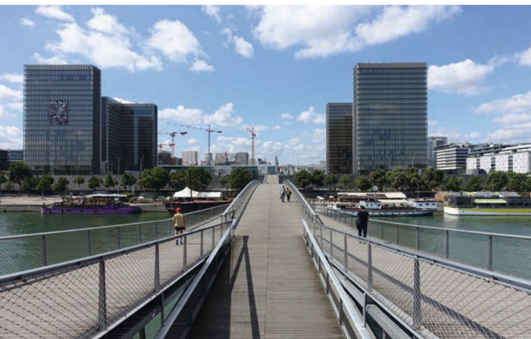
III. 10. Simone-de-Beauvoir footbridge, Paris, France. Photo by G. Vellut, CC-BY-2.0 source: https://commons.wikimedia.org/wiki/File:Passerelle_Simone-de-Beauvoir_@_Seine_@_Paris_(28410220012).jpg#filelinks , (access: 05.02.2024)
