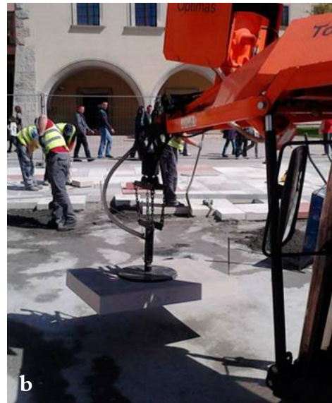
Fig. 3. Road work involving the laying of a stone tile wearing course: a) view of the site, b) self-propelled vacuum lifter with a hydraulic suction mechanism for the transport of stone tiles across the site; all photos by G. Śladowski
