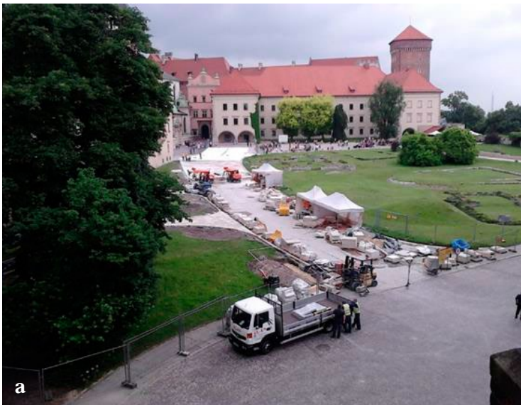
Fig. 3. Road work involving the laying of a stone tile wearing course: a) view of the site, b) self-propelled vacuum lifter with a hydraulic suction mechanism for the transport of stone tiles across the site; all photos by G. Śladowski
