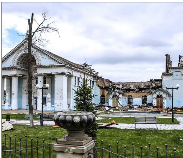
Ryc. 1. Zniszczone dobra kultury w Irpeniu, fot. W. Koskin Fig. 1. Damaged cultural assets in Irpen, photo by V. Koskin
