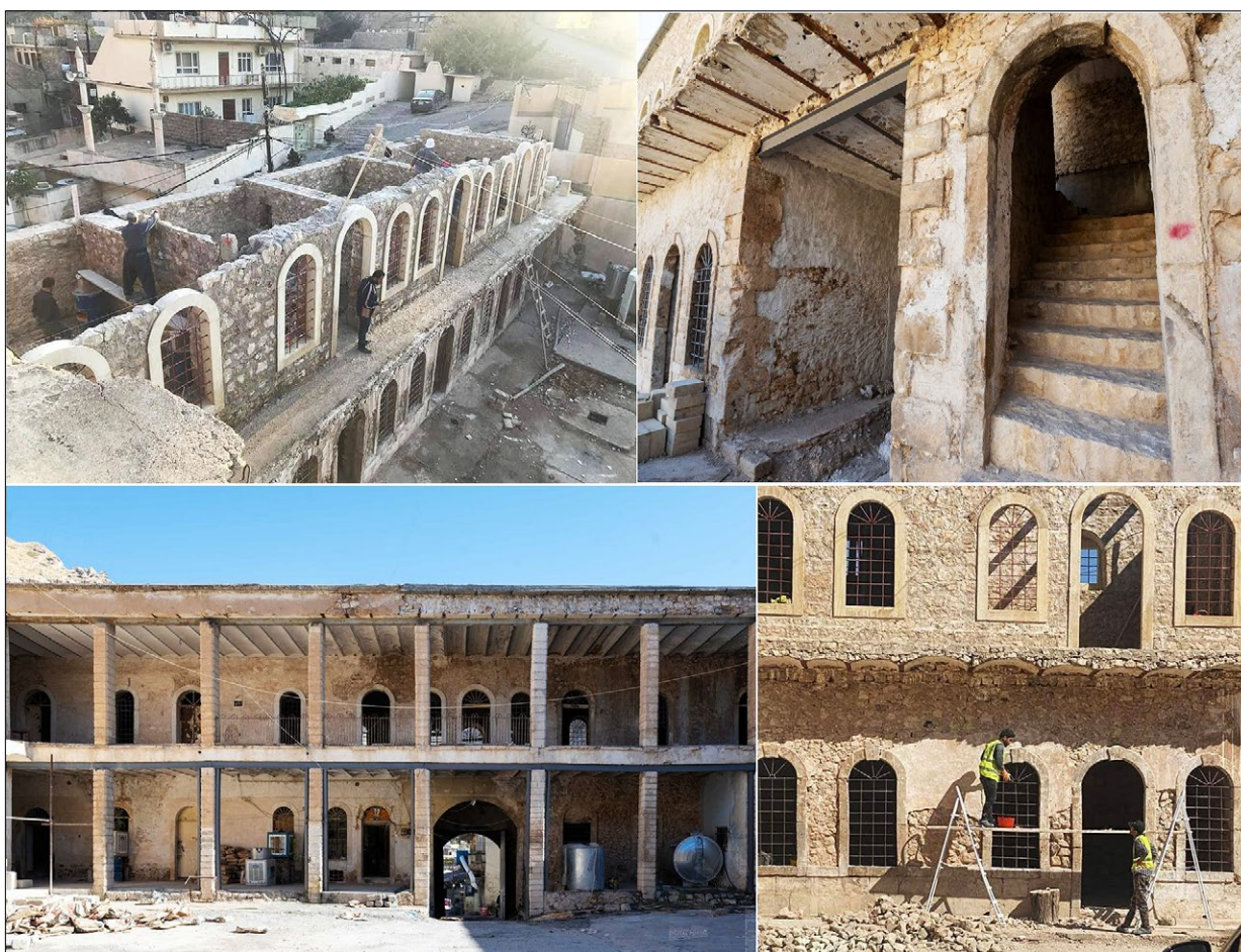
Fig. 5. Preservation work on the Qishla of Akre: a) reconstruction of the first floor walls using traditional materials; source: [pukmedia.com 2022], b) cleaning the original walls, removing the damaged cladding materials, and cleaning the iron beams to prepare them for maintenance work; source: [rudaw.net/ 2023], c) the main entrance facade from the courtyards, showing the scraping of the damaged finishing materials and preparation for restoration work; source: [rudaw.net/ 2023], d) repair work on the walls using tools that are harmless to the original structure; source: [pukmedia.com 2022].
