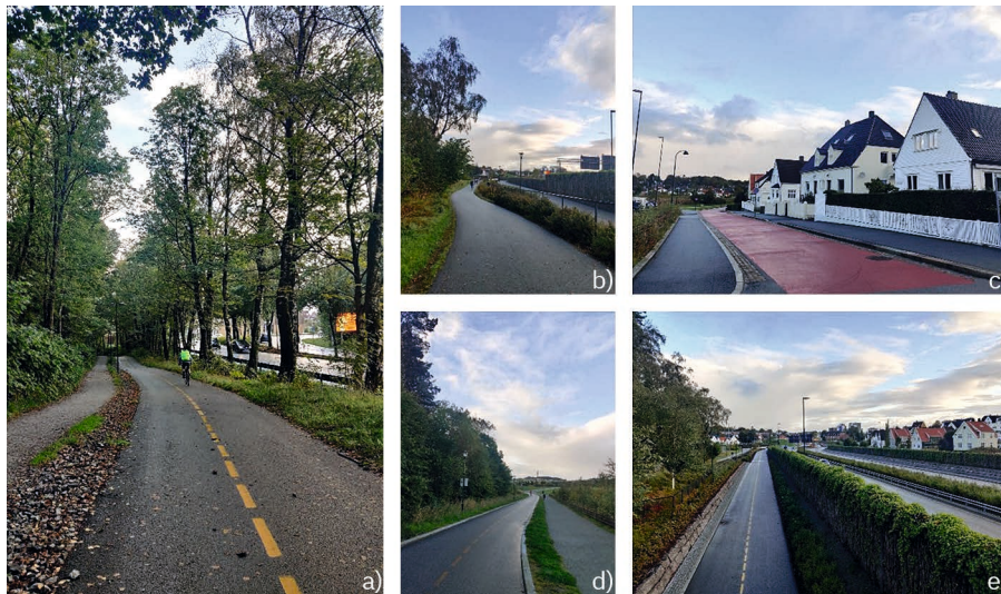
Fig. 5. Conditions of cycling infrastructure in Stavanger: a) cycle path through Mosvatnetparken; b) shared-use roadway for pedestrians and cyclists; c) shared-use roads with priority for cyclists and prohibited parking; d) cycle path through Vålandparken; e) trunk cycle route connecting the municipalities of Stavanger and Sandnes (photo by author)
