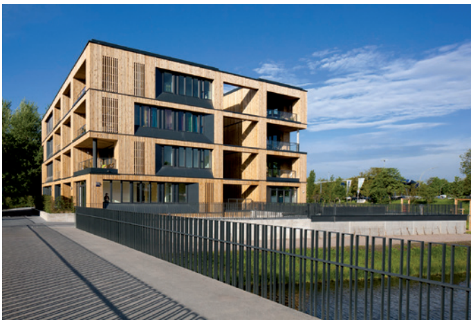
il. 4. The 'Hybrid Development' wooden structure condo (photo courtesy of Bieling Architekten)
