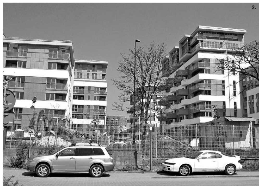
3., 4. New residential city blocks in El Poblenou district in Barcelona.
