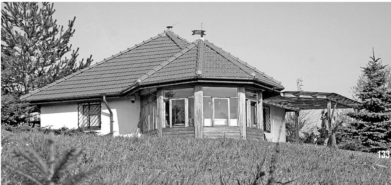
An authorial house “keeping up with” the owners and time, fully modern although beneath the norms.
