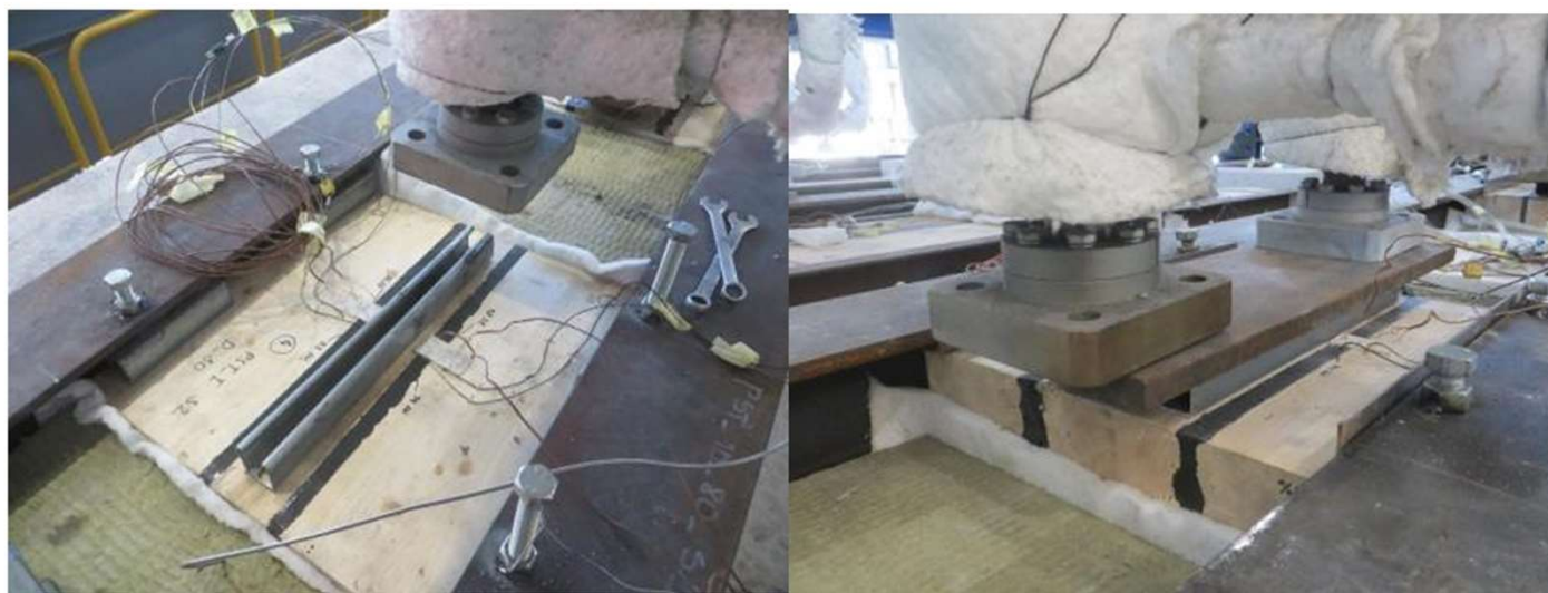
Photo A6.45: Hydraulic jack positioning for mechanical shear loading before the fire resistance test (photo archive, left: 049506d-222, right: 049506d-228)
