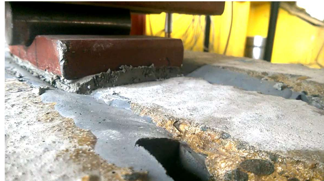
Figure 7: Example of PM polyurethane application
