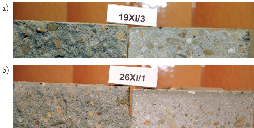
Fig. 3.4. Cross-sections of hardened SCC: a) no segregation, b) severe segregation
