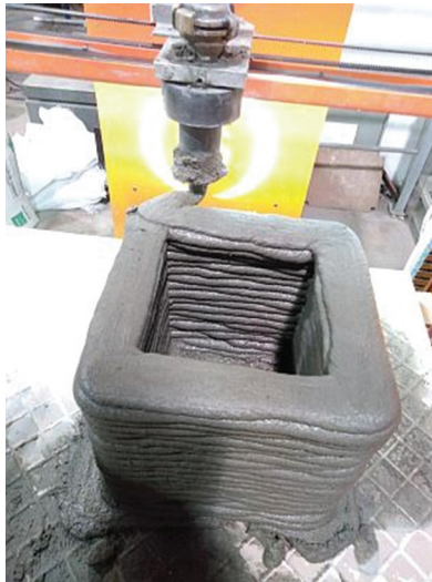
Fig. 5.1. An example of using the Material Extrusion technique to print an element from a concrete mixture
