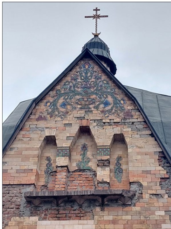
Fig. 7. Current condition of ceramic tile cladding on the eastern facade of the chapel; photo by Y. Ivashko, 2025
