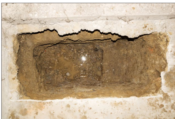
Fig. 6. B-123 concrete foundation; photo by CUT Team
