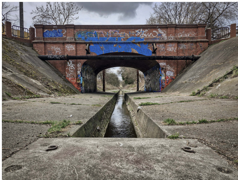
Fig. 2. Concrete-lined channel of the Jasień River near Cieszkowskiego Street – an example of strong technical intervention in the natural structure of the watercourse, 2026. Photo by G. Bajas
