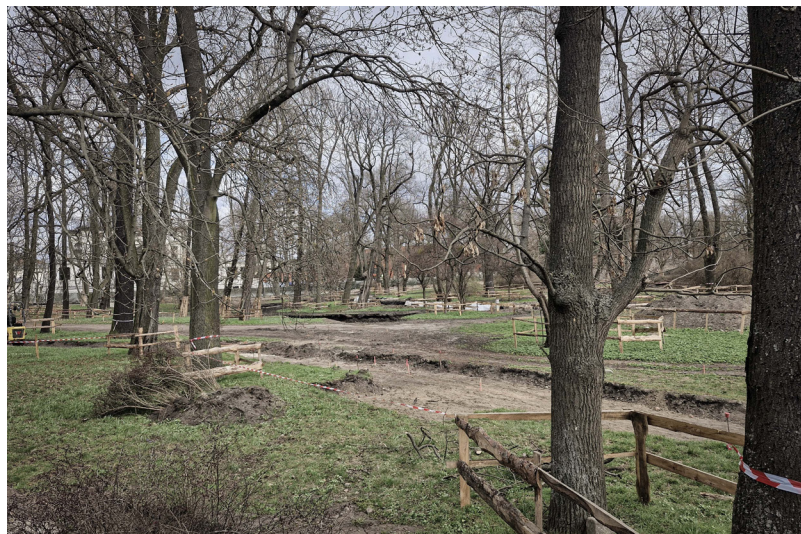
Fig. 4. Reconstruction of the Lamus stream channel – excavation for the new surface section in the park at Kilińskiego Street, 2026. Photo by G. Bajas
