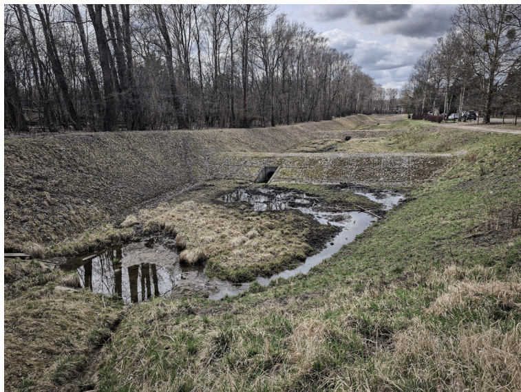
Fig. 5. Varying degrees of channel modification of the Sokołówka River near Fiołkowa Street, 2026. Photo by G. Bajas
