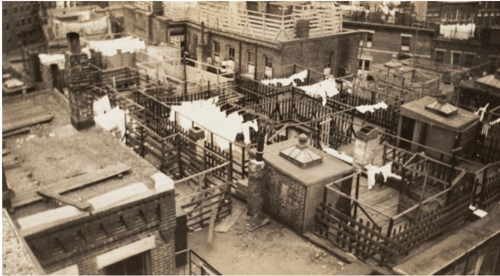
Fig. 1. Apartment block at Cleveland Place, North End (Boston Public Library, 1935)
