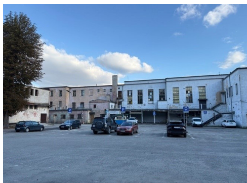
Fig. 7. View from interior of the urban block, 2025. Photo by J. Piątkowski
