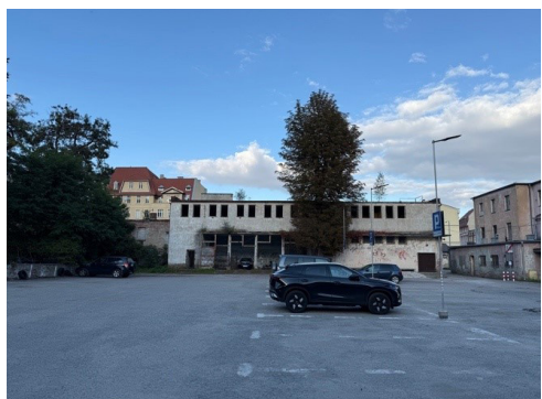
Fig. 6. View from interior of the urban block, 2025. Photo by J. Piątkowski
