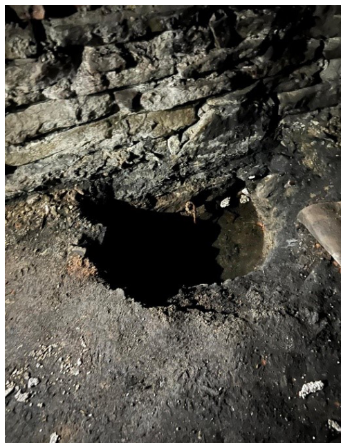
Fig. 9. Executed trial pit, 2025. Photo by author
