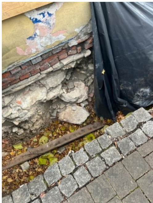
Fig. 7. Fragment of the exposed wall intended for repair, 2025. Photo by author
