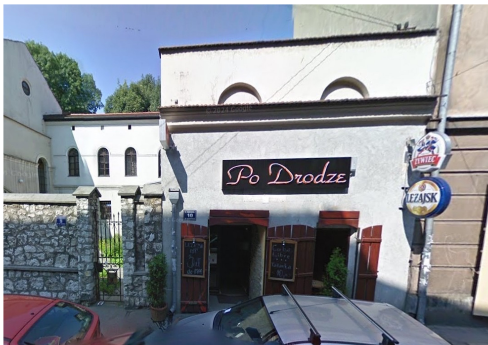
Fig. 16. 10 Warszawera St., September 2009 (Google streetview, 2009)
