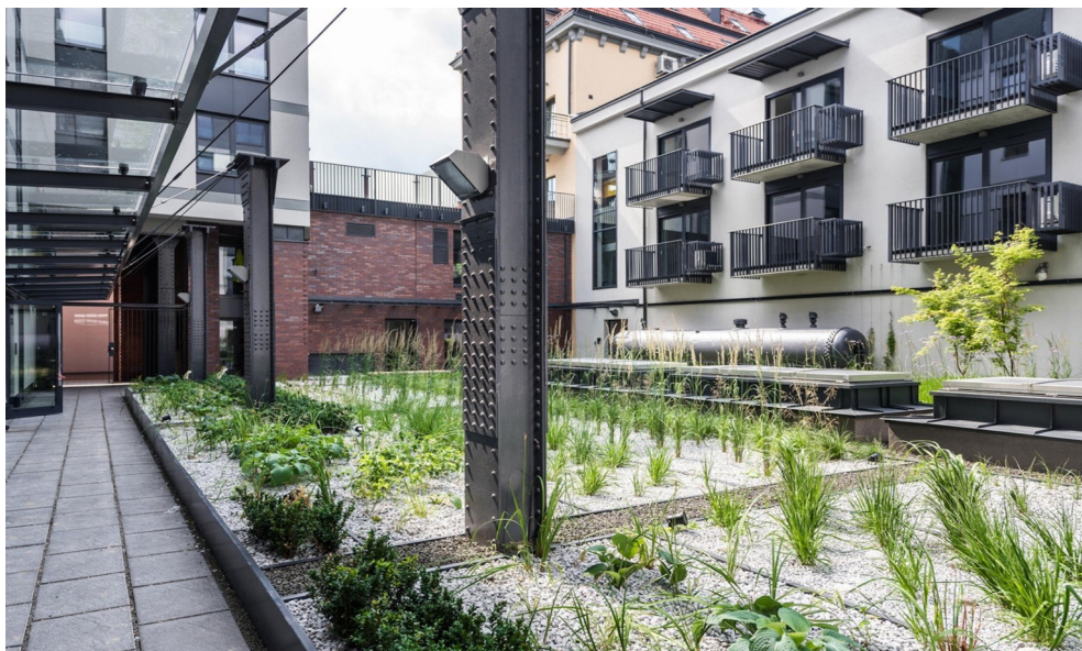
Fig. 7. 21 Św. Wawrzyńca St. Remnants of the building's former use – a steel support structure used to prop up a glass roof (Hamilton May, 2017)
