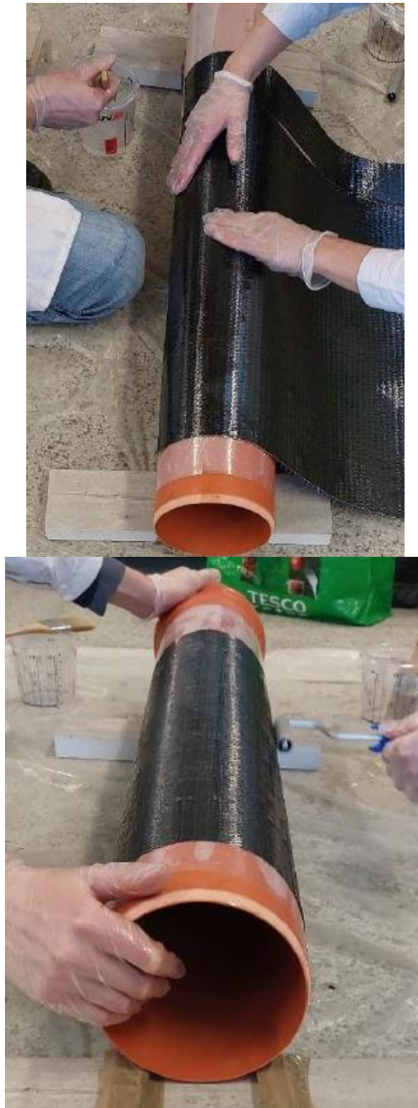
Figure 4. Application and venting of the soaked CFRP.
