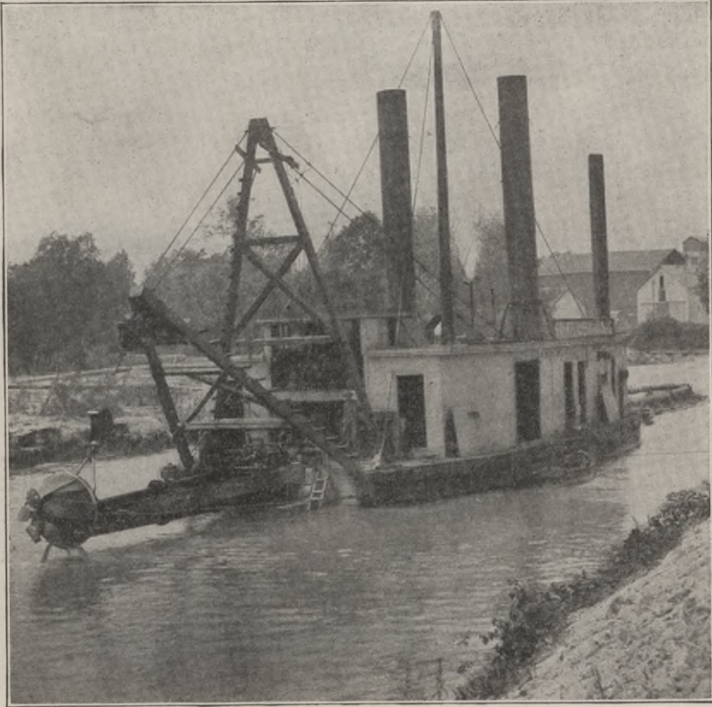
Fig. 61. Typical Hydraulic Dredge on Canal Construction Courtesy of Great Lakes Dredge and Dock Company, Chicago
