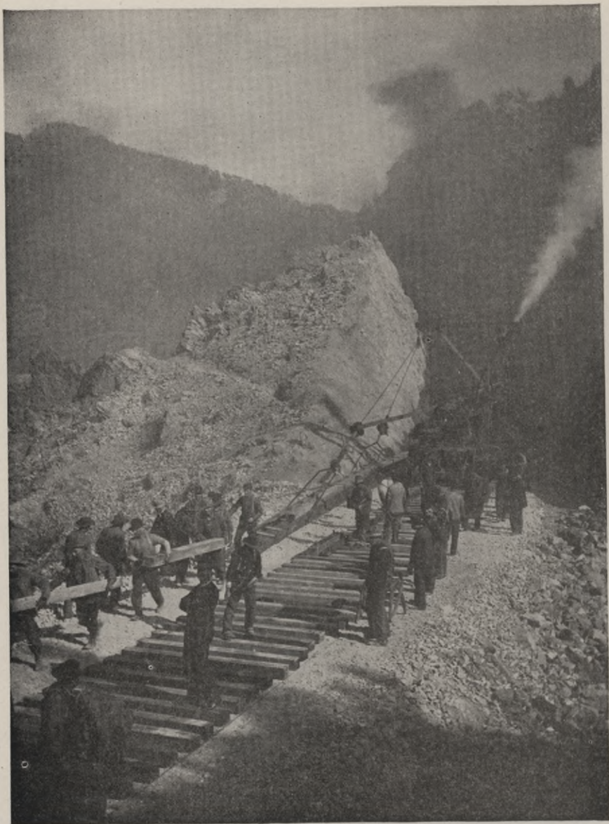
EXAMPLE OF MODERN RAILWAY CONSTRUCTION. TRACK LAYING MACHINE AT WORK
