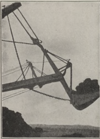
Fig. 42. Dipper and Dipper Handle of Walking Scoop Dredge
