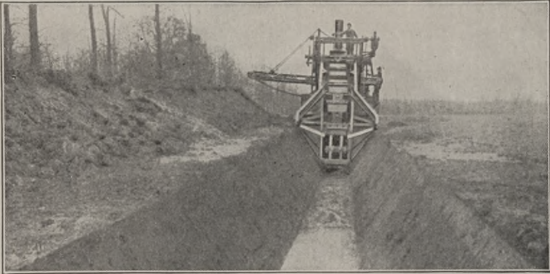
Fig. 37. Wheel Excavator Constructing Small Drainage Ditch
