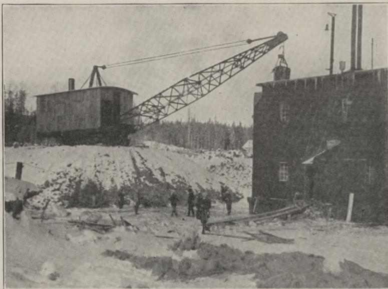
Fig. 32. Drag-Line Excavator Operating on Placer Mine in Siberia
