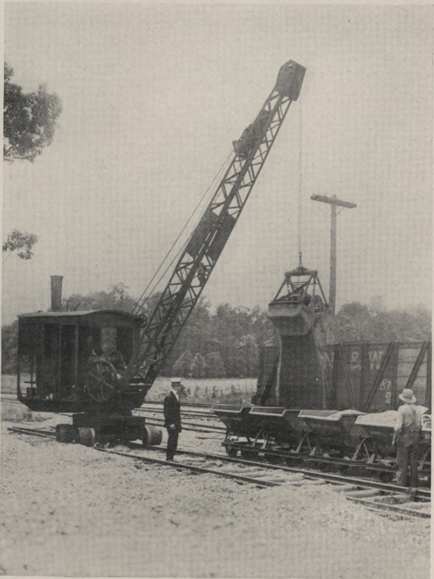
KOPPEL DUMP CARS AND BROWN HOIST HANDLING CRUSHED ROCK FOR CONCRETE ROADS Courtesy of Orenstein-Arthur-Koppel Company, Chicago
